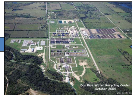
Wastewater Treatment Plant
